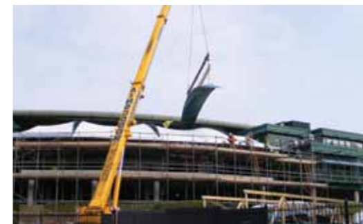
Tension Structures Installation
