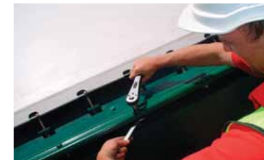
Tension Structures Maintenance and Repairs
